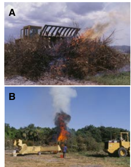
Fig. 14. A, Bulldozer is used to push out and pile up citrus in a commercial grove with citrus canker. Infected and immediately adjacent trees have been previously burned in place to immediately stop the possible dispersal of inoculum. B, Exposed and charred, infected citrus is destroyed by burning.
